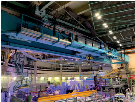
Crane on Level C.
