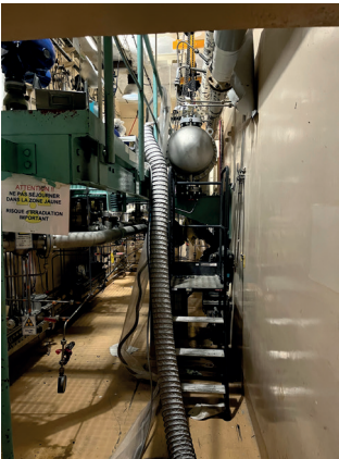
Replacement of B27 heat exchanger.
