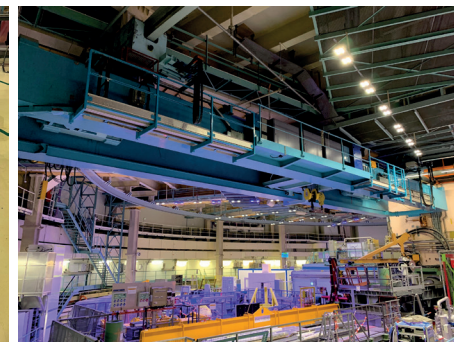
Crane on Level C.
