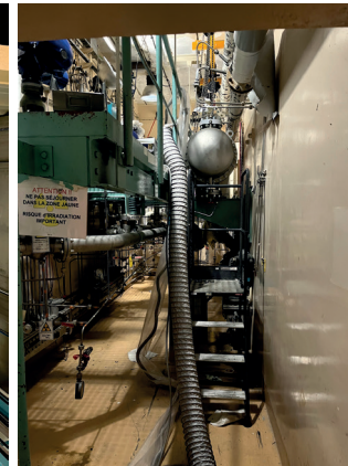
Replacement of B27 heat exchanger.
