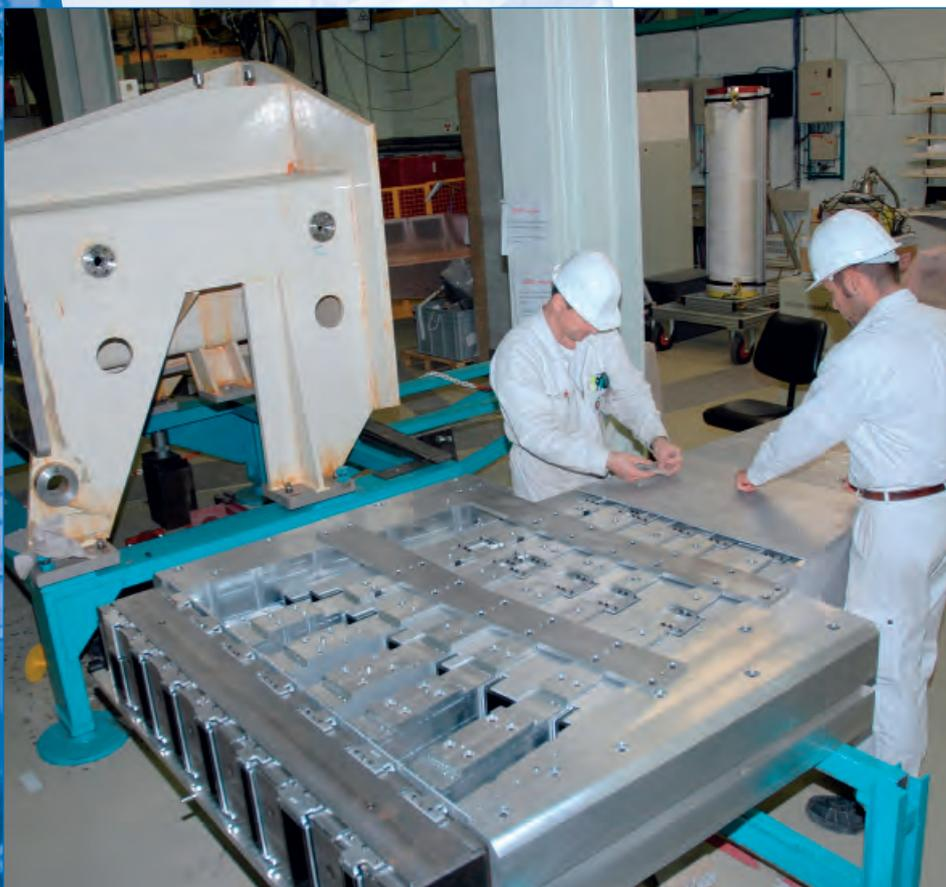
*Figure 1: View of the work to install the new in-pile section of the H1/H2 guides.*
