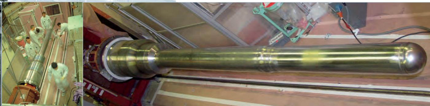
**Figure 1:** The installation of a new zircalloy beam tube thimble, with a life-time well beyond that of the reactor itself - the old aluminium tubes needed to be replaced every 5 - 8 years.
