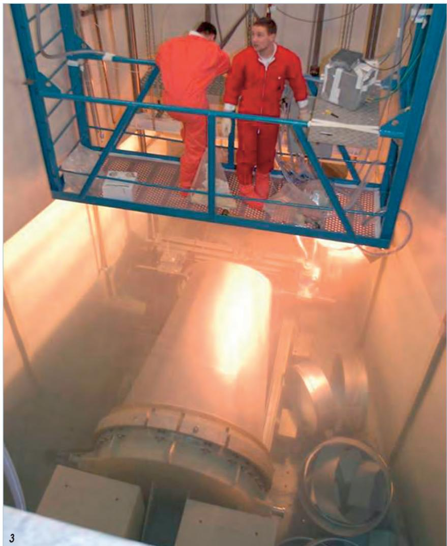
**Figure 2:** When changing the vertical cold source's digital control system, other strategic equipment was also changed or modified, following the lessons learnt over the last 40 years. This is the vertical cold source tank under 18 m<sup>3</sup> of deuterium ballast. It houses the isolation valves and the analysis and conditioning circuits. It is designed to resist a deuterium explosion.
