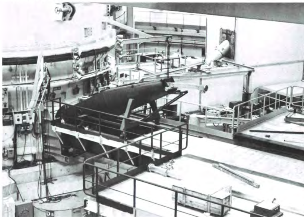
Ultra-cold neutron source during construction
