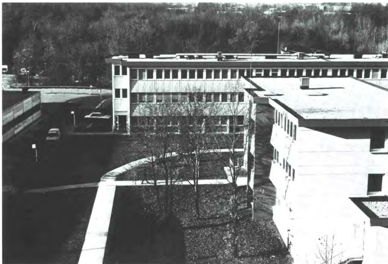
The new computer building completed (right) and the joint biology/EMBL building.
