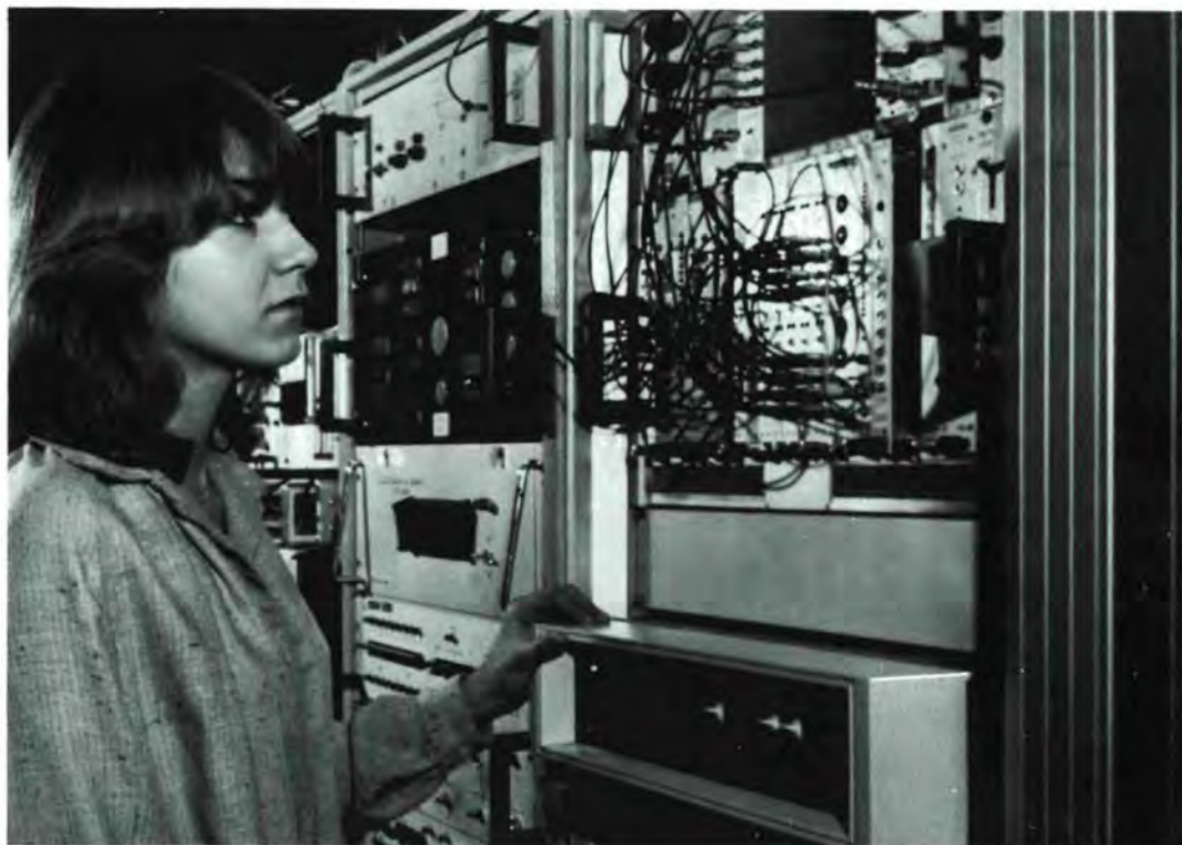
The D1A CARINE replacement (indicated by operator). The Micro-1 computer, manufactured by the British Company "Plessey" is one of the smallest and least expensive parts of the electronics, but uses the same operating system and peripherals as the larger PDP11's.
