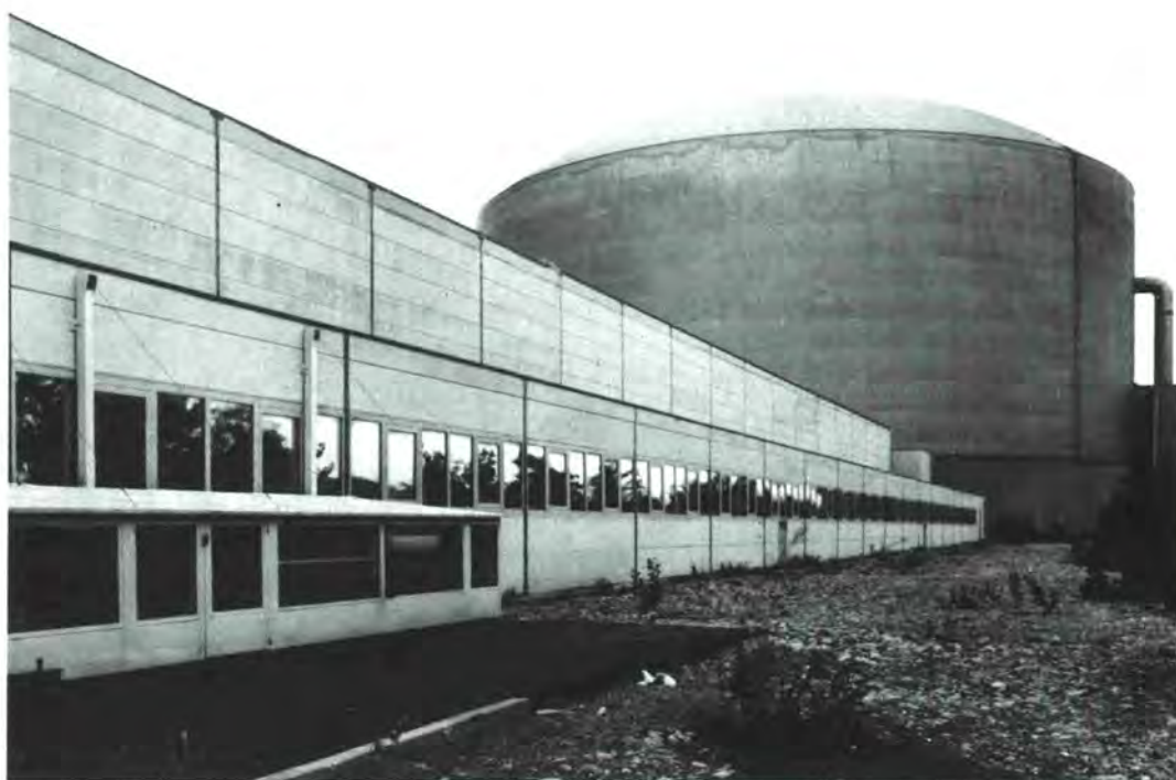
Recent extension to the neutron guide building
