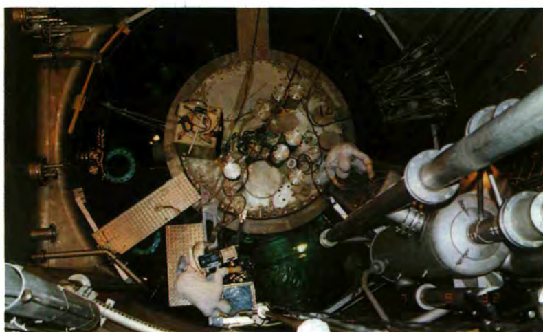
Cutting the H1-H2 beam-tube coupling sleeve in the swimming pool.
