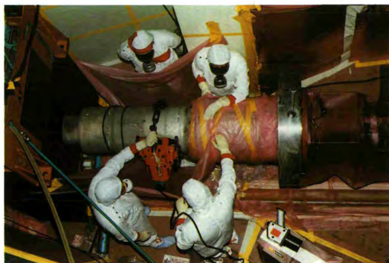
Removal and cutting of the rear part of a liner.
