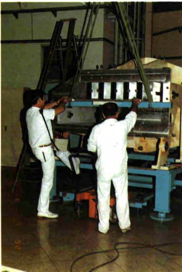
Extraction of the support structure for the cold guides H1 from the housing.
