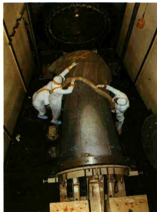
Removal of the H1-H2 coupling sleeve.
