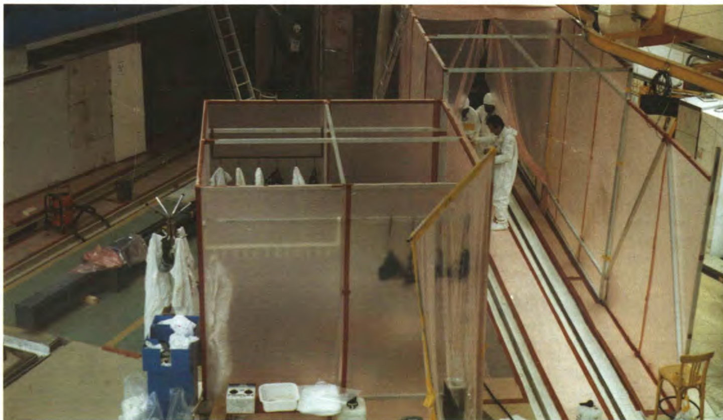
The radioprotective arrangements for the extraction of thimbles. In the picture is the working and dressing area of the technicians.
