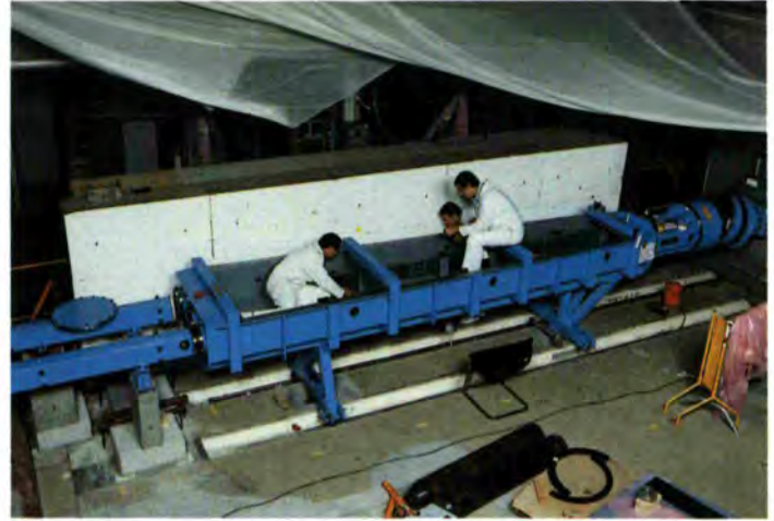
Installation of the neutron guides on the second cold source
