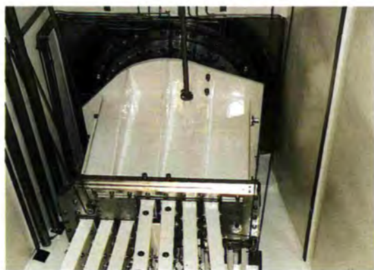
DPT - Fig. 3: The housing of the mechanical support in place on the H1-H2 beam tube. See report p. 128. On the left hand the blanks for the NG12 and NG13 guides, on the right hand the blank of the H18 guide. These guides are not mounted in the out-of-pile part.
