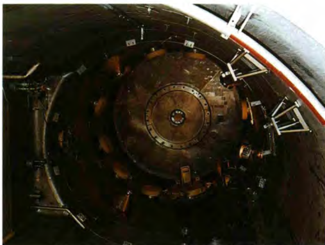
Figure 5 shows the swimming pool prior to the installation of the vessel. Note the covered channels through the reactor pool - the coupling sleeves that will contain the beam tubes will be moved in through these channels and connected to the vessel.
