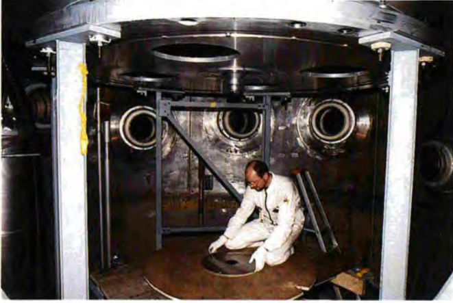
Figure 8 shows the bottom of the vessel placed on supports with a template used to adjust the sleeve with respect to the vessel axis. Figure 9 shows the same sleeve undergoing leak tests just after welding.
