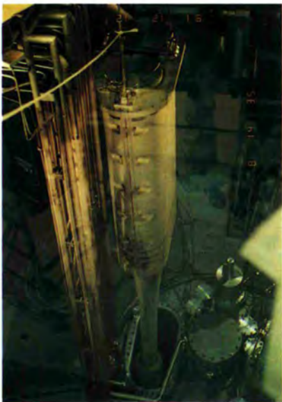
Underwater removal of the beam-tube for the spectrometer PN2 (BILL).
