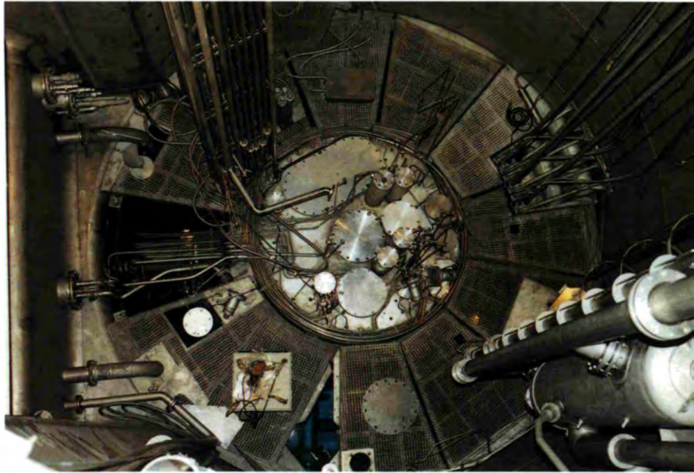
The same view with all in-pile units removed.
