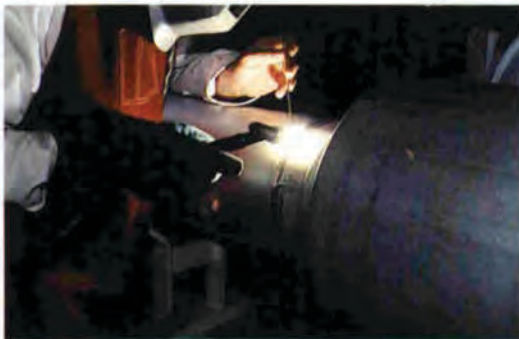
Fig. 10b: Close-up of the welding procedure.
