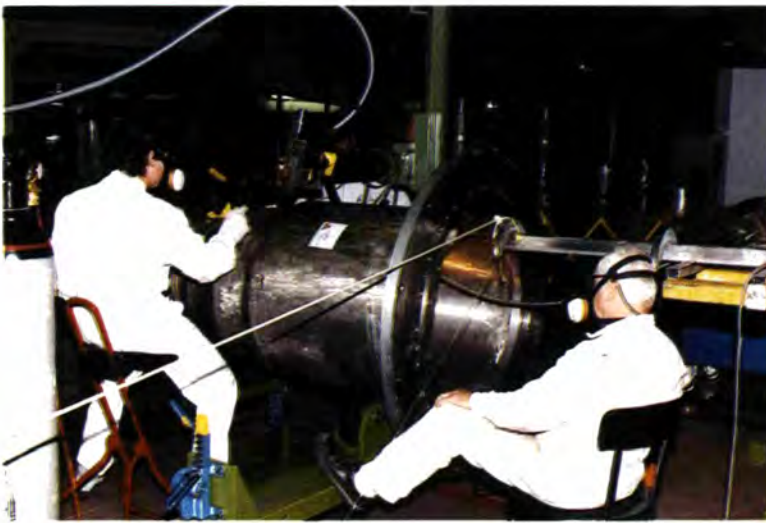
Fig. 15: A new stainless steel bellows is welded to the outer part of the beam tube by S. Müller and F. Müller.
