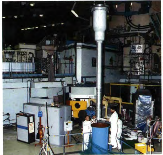
Fig. 8: A beam tube thimble under leak test. J.F. Garin-Cuchet, J. Pellegrino, J.P. Gonella, C. Yoccoz.
