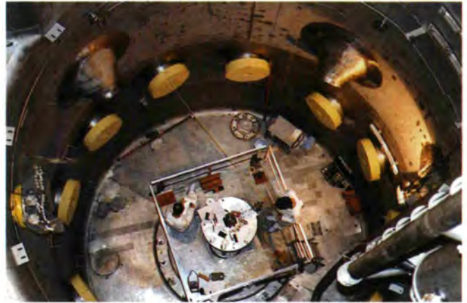
Fig. 20: Geometrical checks on the beam tubes by F. Saint Suplice and G. Signoretti.
