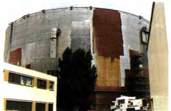
Fig. 18: Repainting of the reactor shell.
