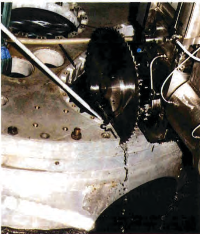
Fig. 3: The cutting machine attacks the upper part of the reactor vessel.
