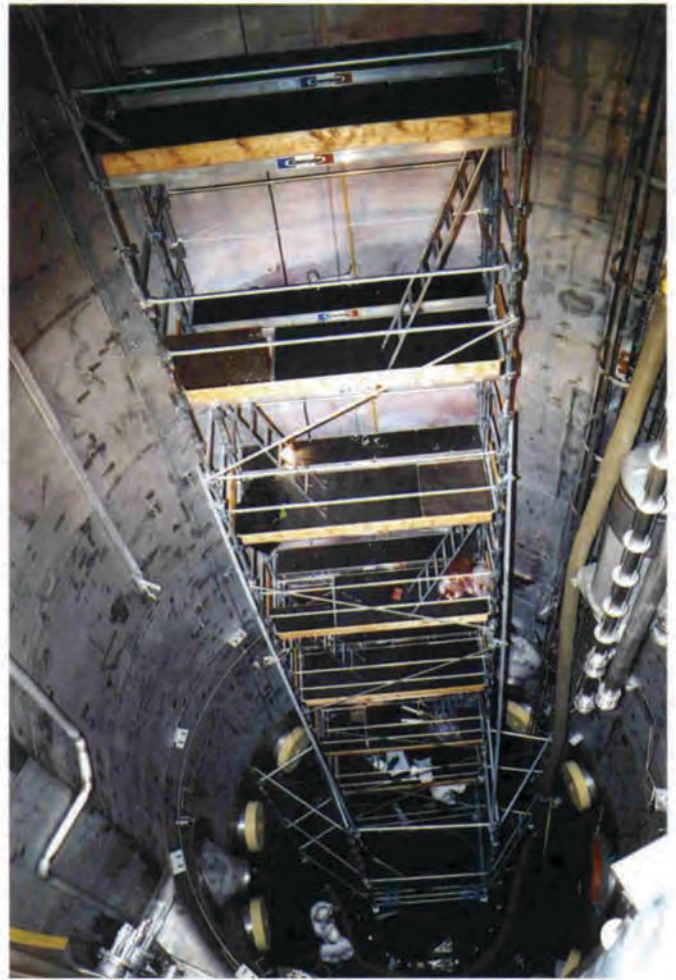
Fig. 11: The swimming pool lining under inspection.
