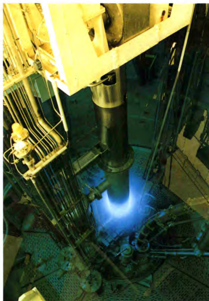
Fig. 1: Unloading the fuel element from cycle 99.
