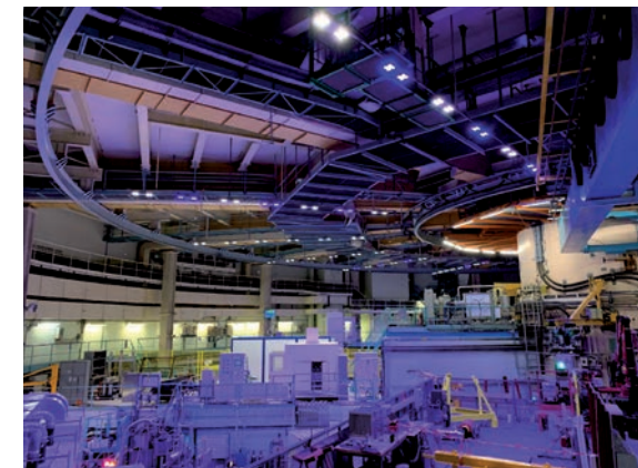
Installation of a fire sprinkler system on Level C.
