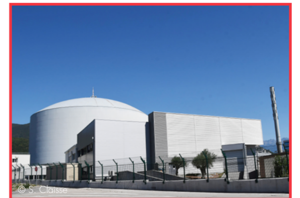
From top: Getting ready for the replacement of the H4 beam tube. The outcome of the 10-year safety assessment authorises the ILL to operate for the next ten years. The Reinforcement of Physical Protection (RPP) project – launched in 2017 – will be finalised in 2021.
