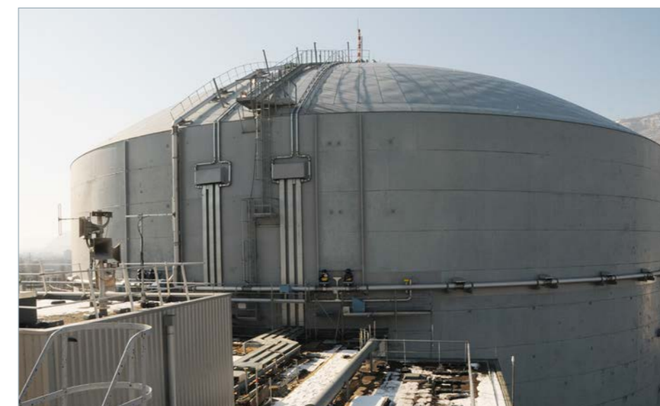
Part of the reactor's outer shell with the new seismic depressurisation circuit, shell penetrations, and cableways linking the reactor to the new seismically resistant electronics room.
