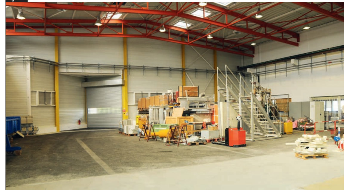
Current state of the almost empty guide hall ILL22.
