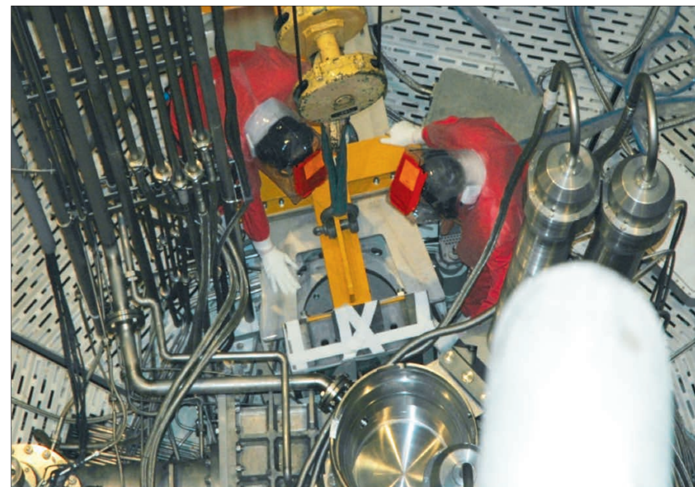
Inserting the CRU (emergency reflood circuit) into the reactor vessel.
