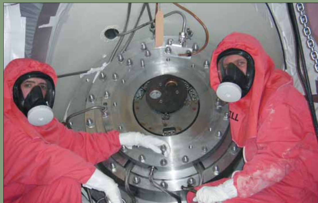
Preparing the removal of the IH4 beamtube.
