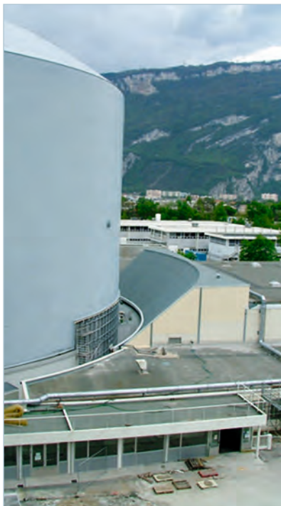
Figure 1: View of the separation between the reactor building and one of the guide halls.
