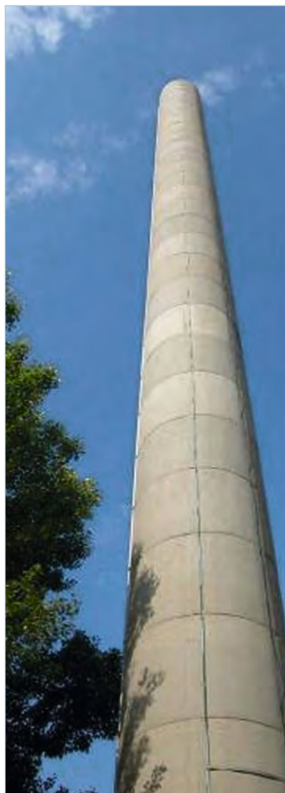
The reactor chimney resistance in case of seism was also tested.
